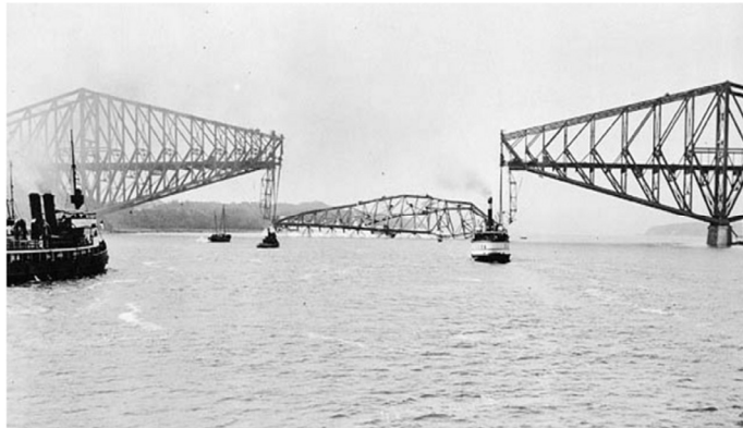
1916 hoisting failure
