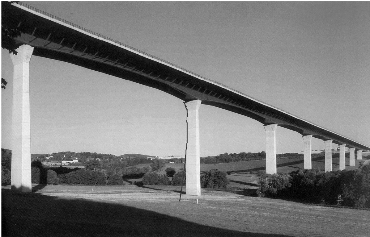
Reichenbach Valley Bridge, 2003 Eng. Büro Peter + Lochner
