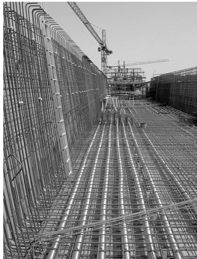
Reinforcement of Weidatalbrücke
