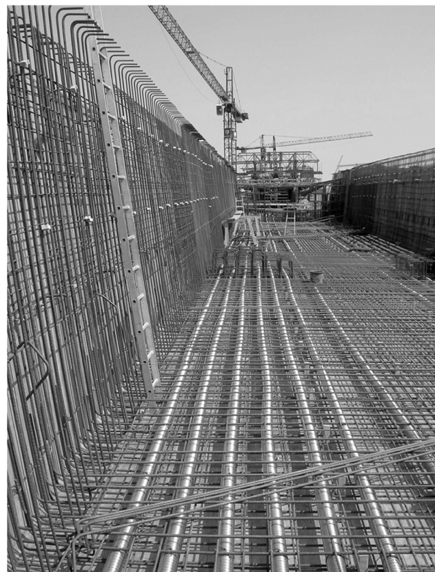
Reinforcement of Weidatalbrücke
