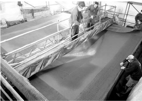
Figure 13: Manufacturing of the TRC hyper-shell layer by layer by shotcrete [photo: © RWTH Aachen], [38]
