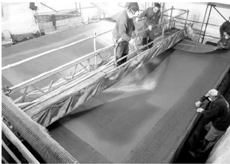
Figure 13: Manufacturing of the TRC hyper-shell layer by shotcrete [photo: © RWTH Aachen], [38]
