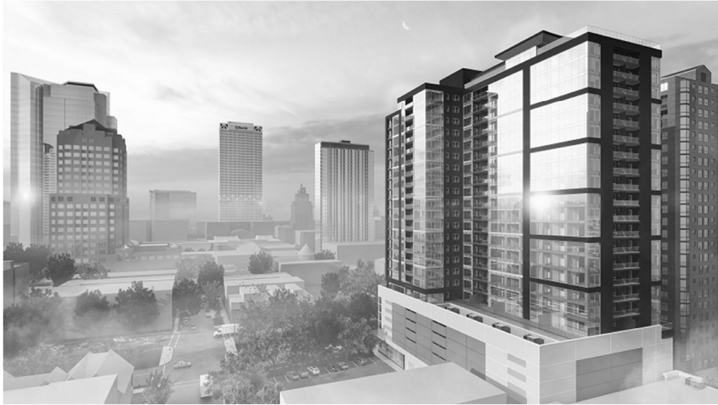
Ascent in Milwaukee – 25 stories, under construction
