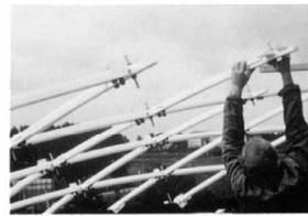
6.16 Assembly of the grid elements
