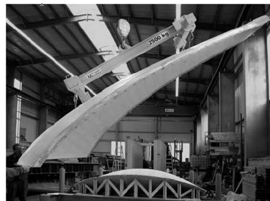
Figure 10: Demolding of a hardened shell element in the concrete yard in Kahla/Saxony [photo: Daniel Ehlig, TU Dresden]
