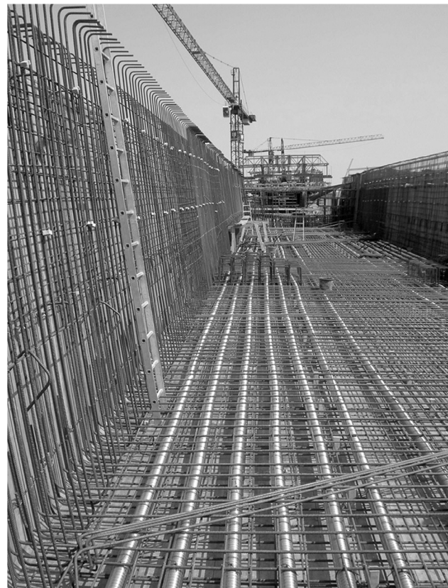
Reinforcement of Weidatalbrücke
