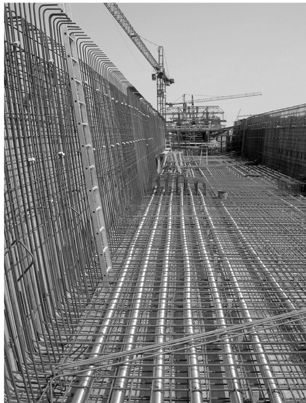
Reinforcement of Weidatalbrücke
