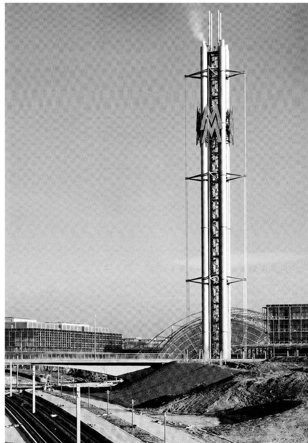
Messe Leipzig – Cable braced tower. Jörg Schlaich
