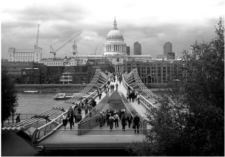
Millennium Bridge, London Foster and Partners + Arup
