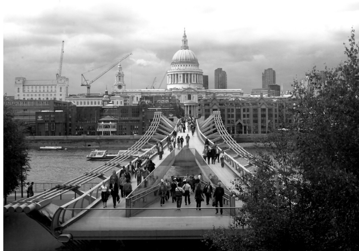
Millennium Bridge, London Foster and Partners + Arup
