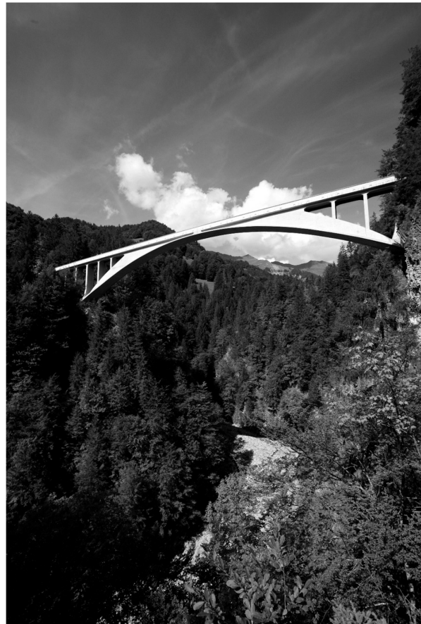
Salginatobel Bridge Switzerland, 1930 300 ft span 42 ft rise Robert Maillart
