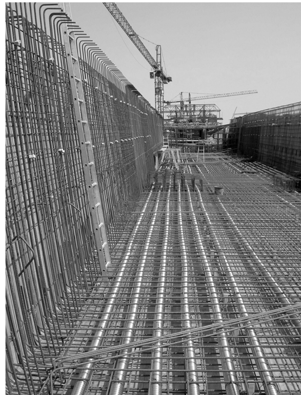
Reinforcement of Weidatalbrücke photo by Störfix
