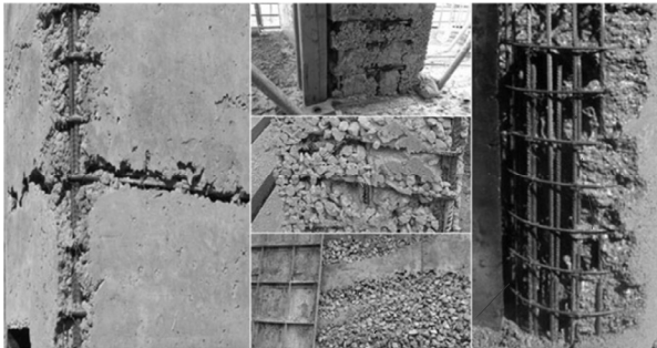
https://www.constructioncost.co/honeycombing-in-concrete.html
