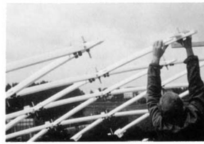
6.16 Assembly of the grid elements
