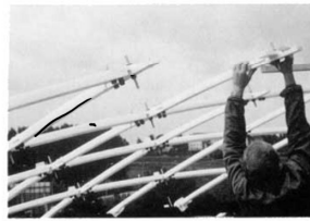
6.16 Assembly of the grid elements
