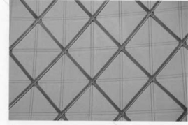
6.18 A segment of the grid showing the double pattern formed by the slats and cables
