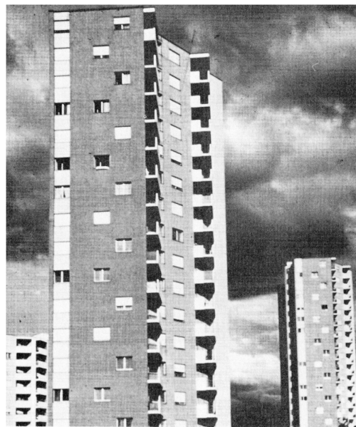
Figure 17.1 16-story loadbearing brick masonry building, Biel, Switzerland. (Courtesy of Brick Institute of America.)
